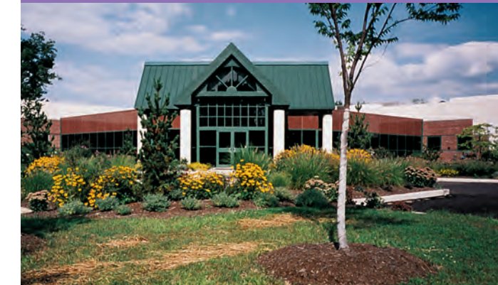
FOREST PARK WATER TREATMENT FACILITY
