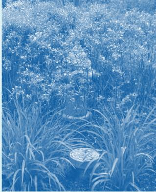
The North Wales Water Authority abides by the International Fire Codes and section 508.5.4 states that posts, fences, vehicles, growth, trash, storage and other materials or objects shall not be placed or kept near fire hydrants and that fire departments shall not be deterred or hindered from gaining immediate access to fire protection equipment or fire hydrants.
