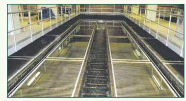
Sedimentation basin with inclined plates
